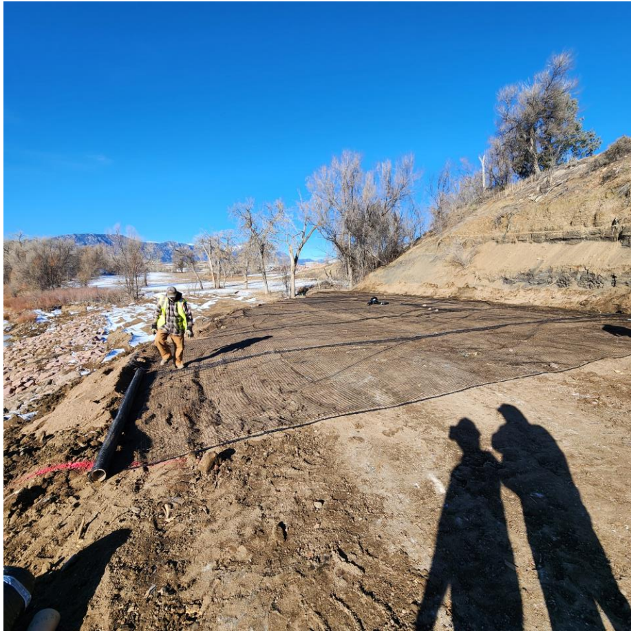
Installation of geogrid
