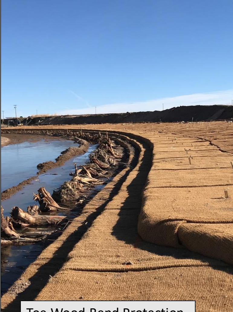
Toe Wood Bend Protection (FCWD/Matrix Project)
